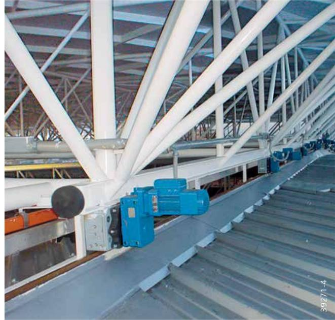
Furthermore, the patented torque bracket enables torque to be transmitted from the geared motor to the wheel block without any radial force. This reduces the load on the drive shaft and extends its service life.
