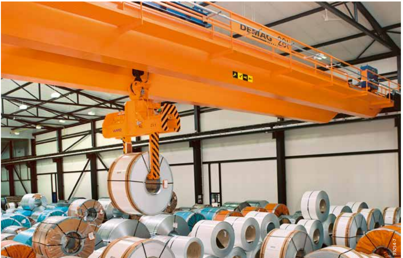
Careful handling of steel strip in a coil store
