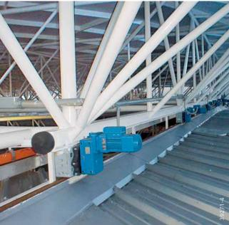
Furthermore, the patented torque bracket enables torque to be transmitted from the geared motor to the wheel block without any radial force. This reduces the load on the drive shaft and extends its service life.
